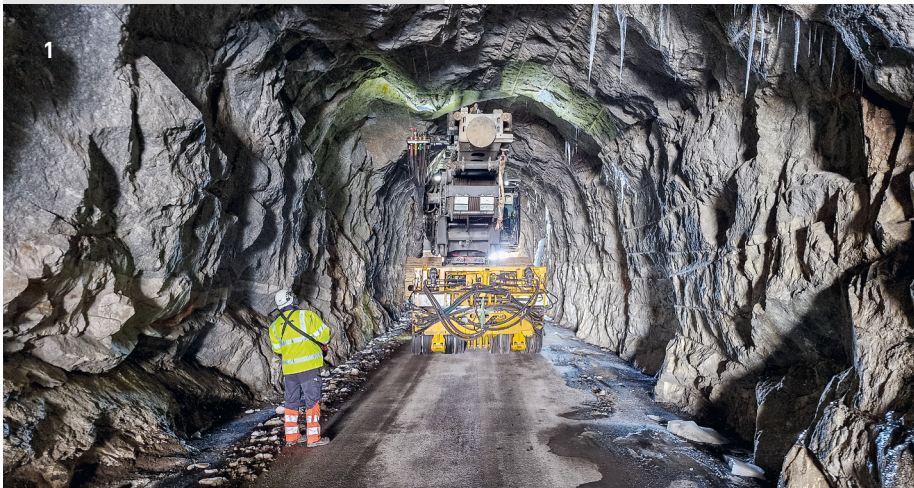
1 Some of the construction machinery had to be transported to the site along narrow roads with steep gradients. © ZÜBLIN / 2 The bored piles were fabricated with centimetre precision. © ZÜBLIN
