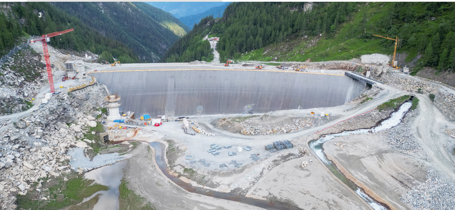
3 The rock-fill dam is being raised by seven metres. © STRABAG
