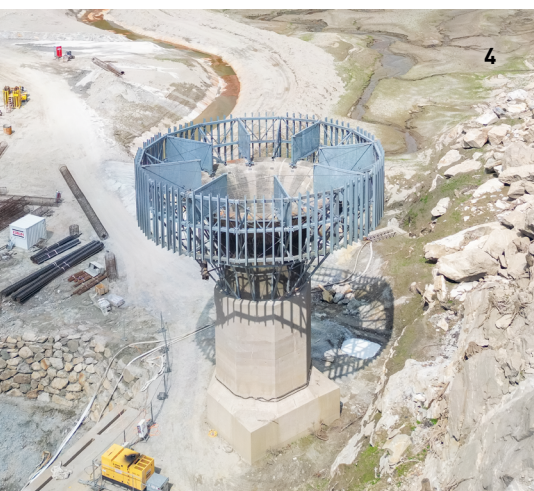
4 The flood funnel is used for flood protection. © STRABAG / 5 The Wurten Reservoir seen from above. © ZÜBLIN
