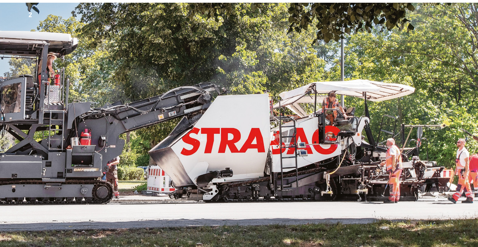
2 Installation of ClAir® Asphalt with the innovation paver and hopper in Erlangen. © STRABAG AG/ 3 The first ClAir® Asphalt pilot project in April 2019 at Neckartor in Stuttgart © STRABAG AG/Thomas L. Fischer
