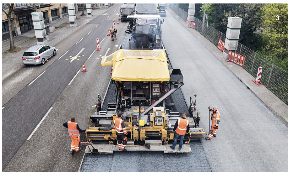
2 Installation of ClAir® Asphalt with the innovation paver and hopper in Erlangen. © STRABAG AG/ 3 The first ClAir® Asphalt pilot project in April 2019 at Neckartor in Stuttgart © STRABAG AG/Thomas L. Fischer
