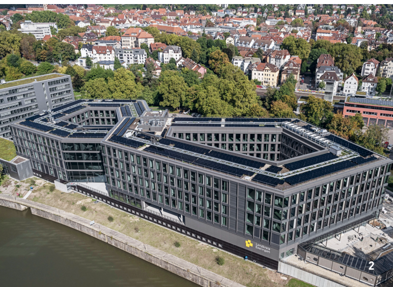
2 New Construction on the Neckar: The sustainable and resource-efficient construction of the new Esslingen District Office using recycled concrete was based on a circular construction concept. © Ed. Züblin AG / Niels Schubert
