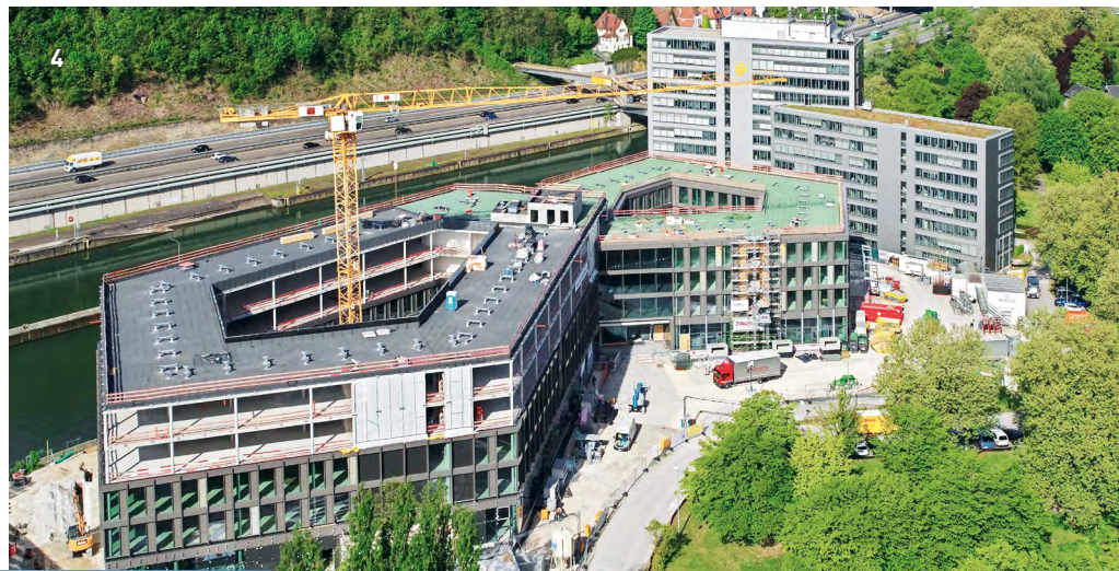
4 The new district administration building was constructed using a high proportion of recycled building materials. © Esslingen district / 5 More than 90 percent of the building materials from the demolition of the original 1978 building are being recycled. © Landratsamt Esslingen, Andrea Wangner
