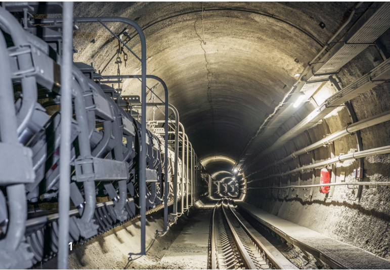
1 Tunnel with conveyor belt, track and pedestrian pathwa / 2 Train loadout
