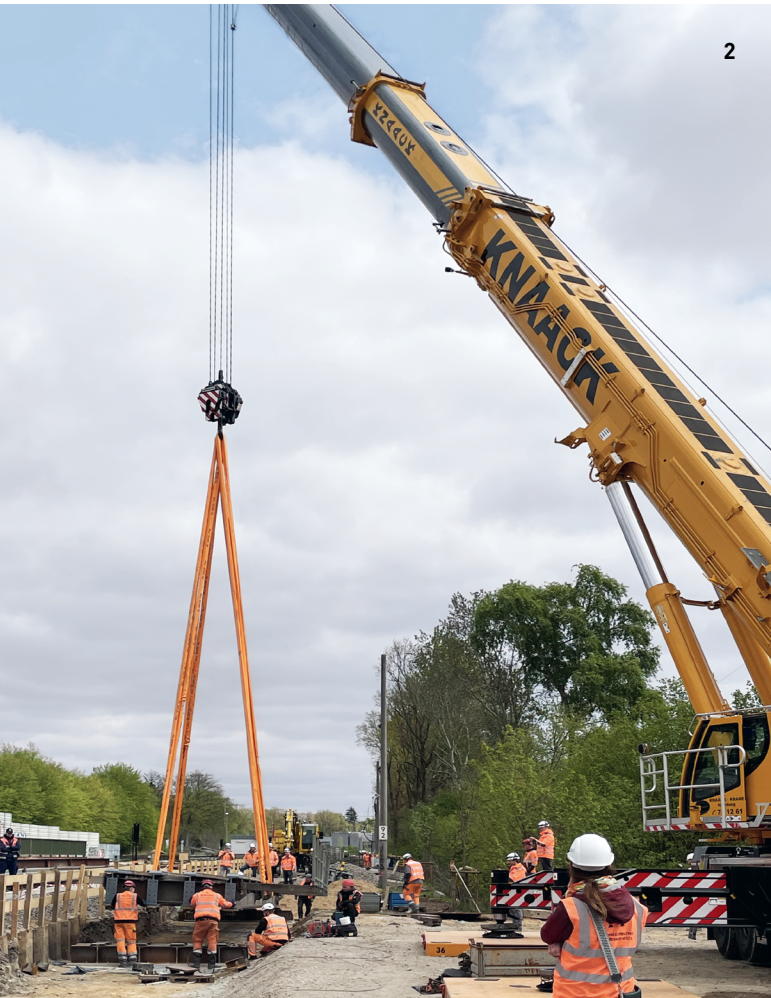
2 Lifting-in of the temporary bridges for the start of construction on the U5's Sengelmannstraße station by the consortium of ZÜBLIN and Wayss & Freytag © HOCHBAHN
