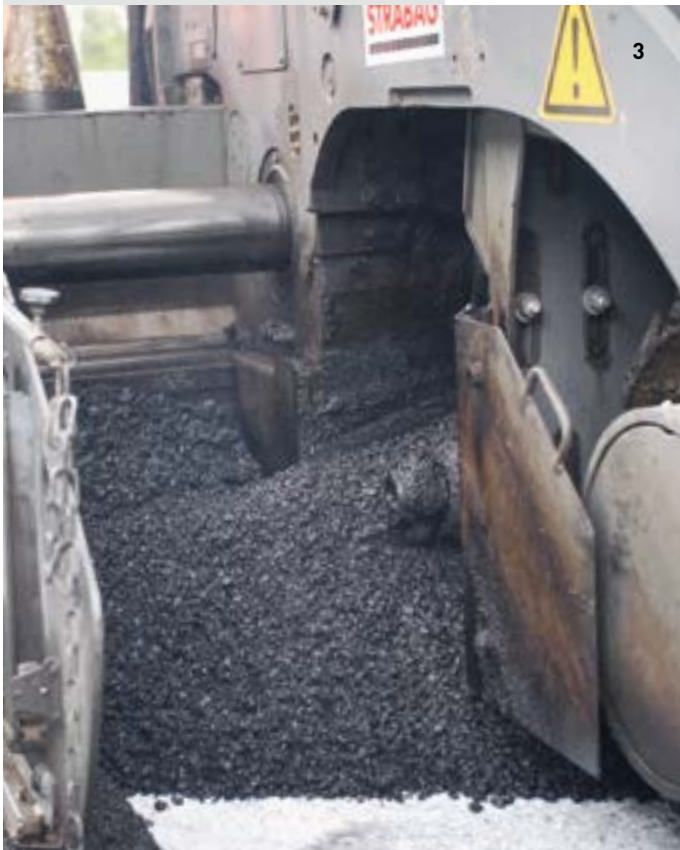
3 The mix for the A1's base layer contains 40 percent recycled asphalt – significantly more than usual. © Sebastian Sieberer
