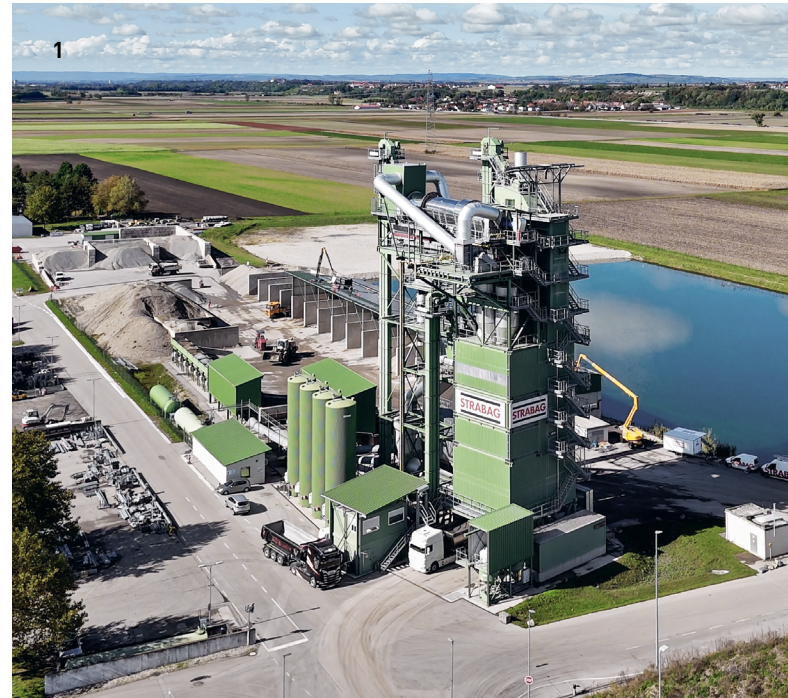
Cover: The mixture on the A1 contains a high proportion of recycled asphalt. / 1 The STRABAG asphalt mixing plant in Hausleiten is very modern. / 2 For Axel Thomaschütz (STRABAG AG Austria), asphalt recycling is a key to making road construction more sustainable. © Sebastian Sieberer
