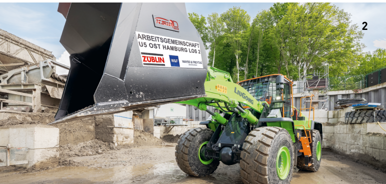
2 For soil management on the construction site, the project team in Lot 2 is using a zero-emission electric wheel loader. © Ed. Züblin AG, Sebastian Engels Fotografie / 3 Lifting of fully assembled rebar cages by crane at the U5 construction site in northeastern Hamburg. © Ed. Züblin AG, Sebastian Engels Fotografie
