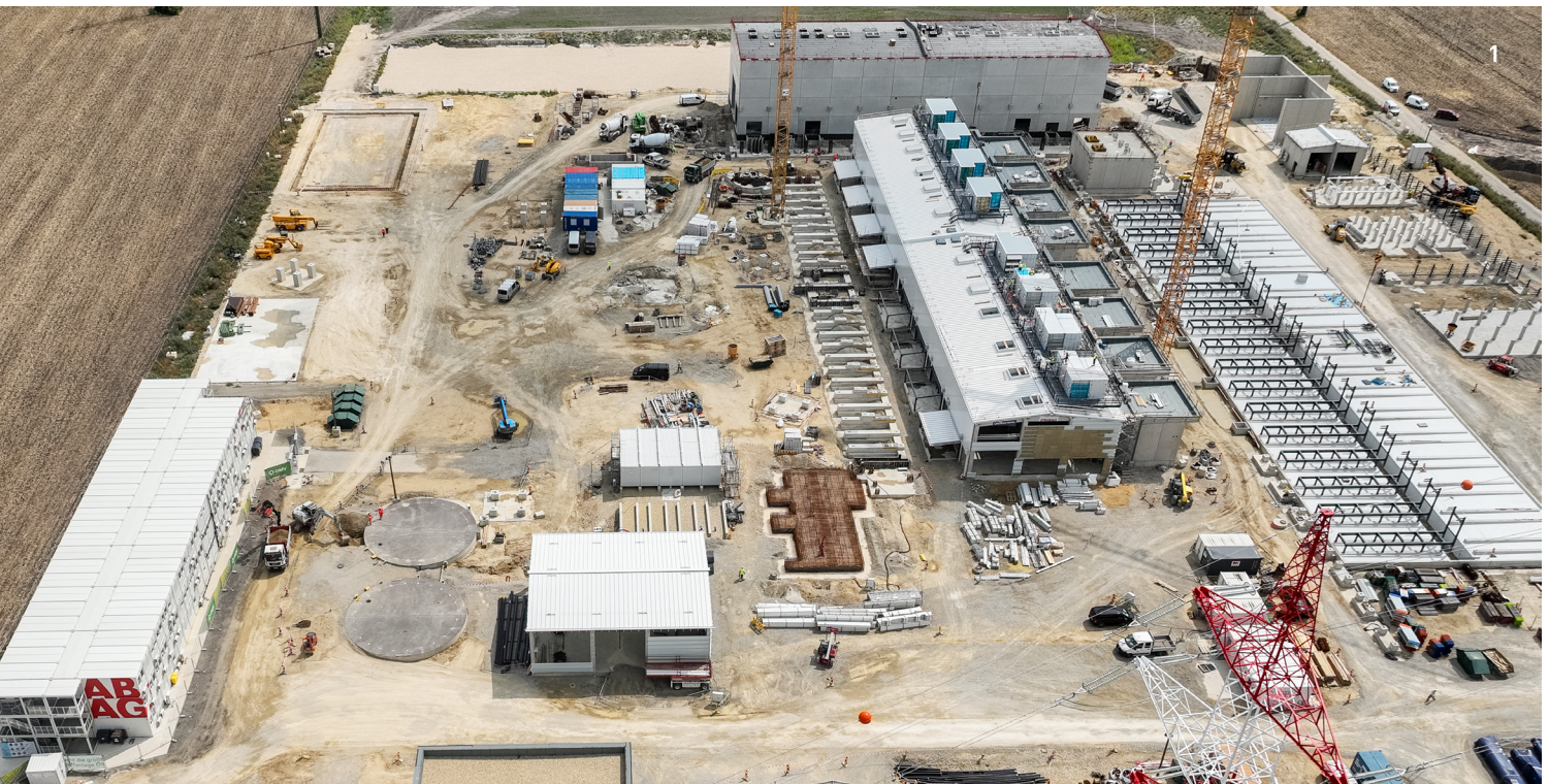
1 Austria's largest electrolysis plant is being built in Bruck an der Leitha. © STRABAG
