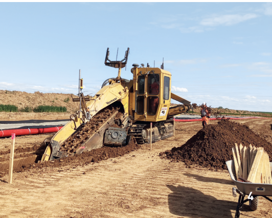
4 Milling instead of excavating on SuedLink: STRABAG combines the use of a trench milling machine with backfilling using liquid soil for the route construction in Unterfranken. © STRABAG AG / 5 Two or more regional STRABAG units often join forces for route construction projects. © TenneT Germany
