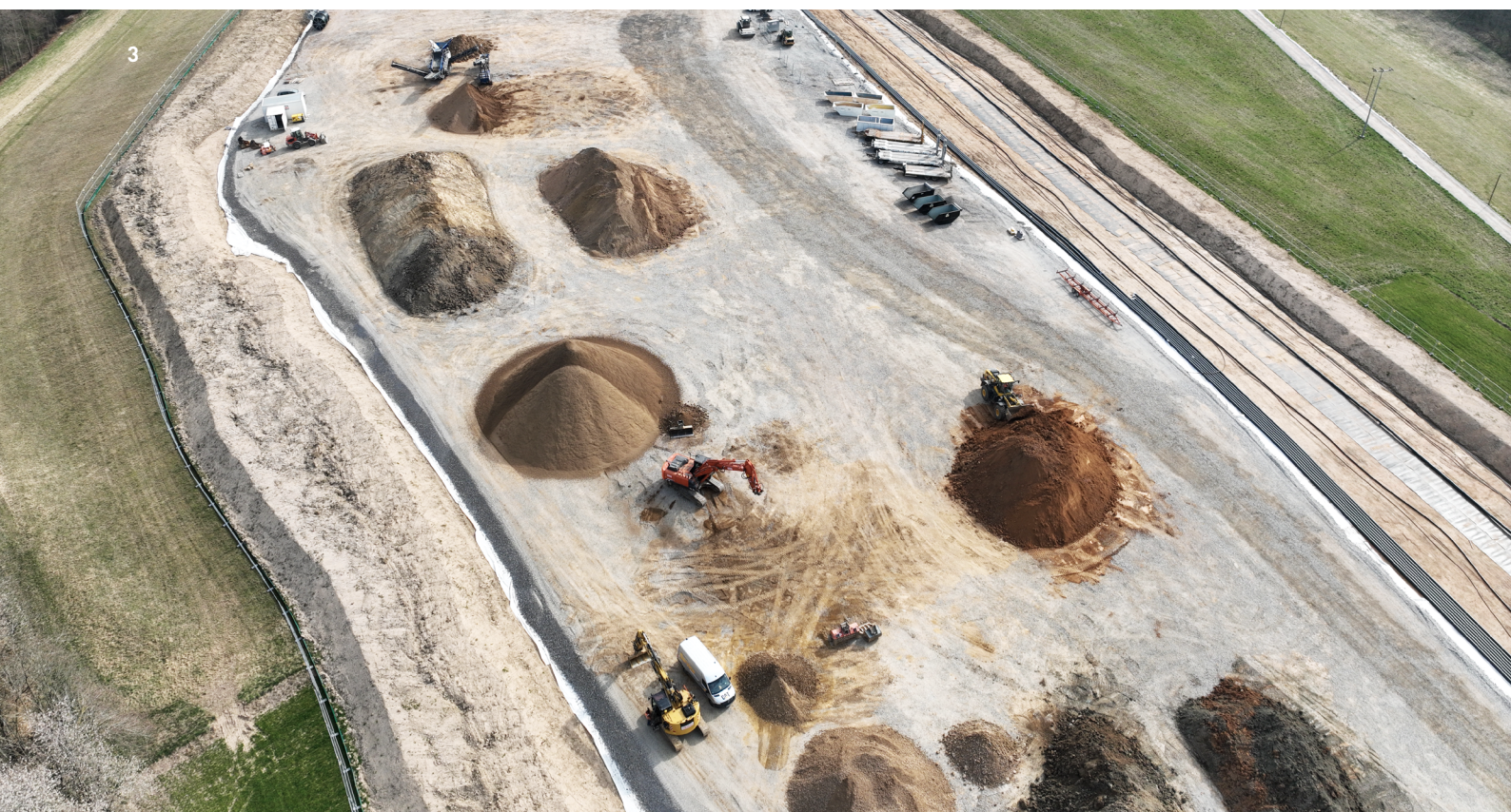
3 STRABAG carefully separates the excavated soil layers and specifically improves the thermal conductivity of the layer close to the pipes before reusing it to backfill the trenches. © STRABAG AG
