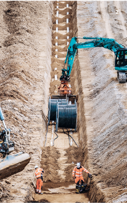
2 Earthworks on a massive scale: up to 60 excavators and 36 wheel loaders are in use every day for the construction of the SuedOstLink section in the Oberpfalz. © TenneT Germany
