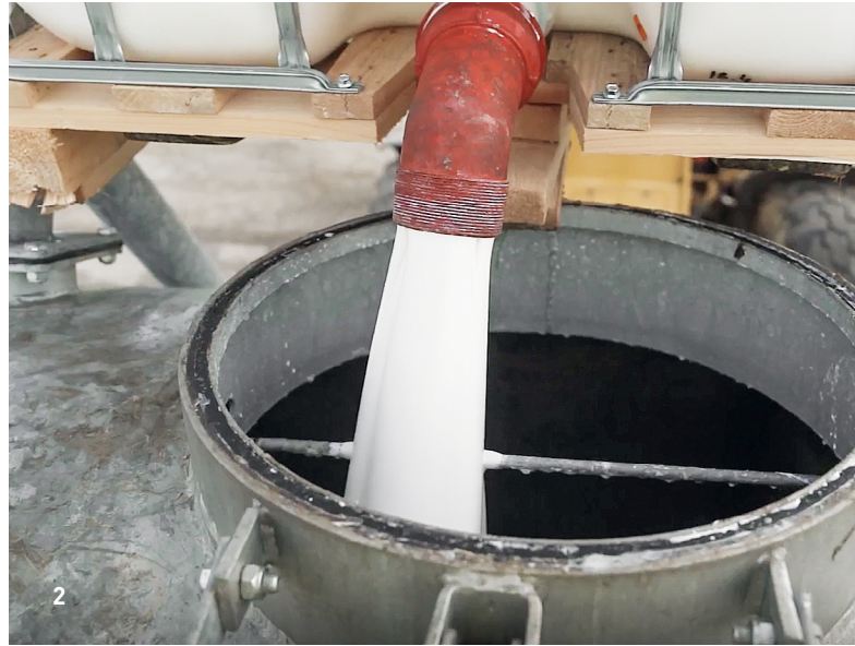
2 The polymer binder is individually dosed, mixed with cement into the building material mixture and then compacted. © Gert Beer
