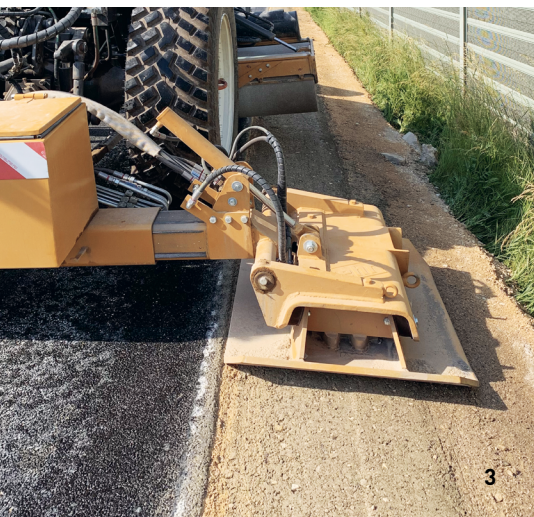
3 Road shoulders can be rehabilitated using polymer binders without material replacement. © Andreas Fuchs/STRABAG
