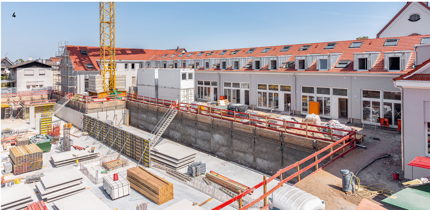
4 The confined conditions on a refurbishment site call for sophisticated construction logistics. © Henning Kretz
