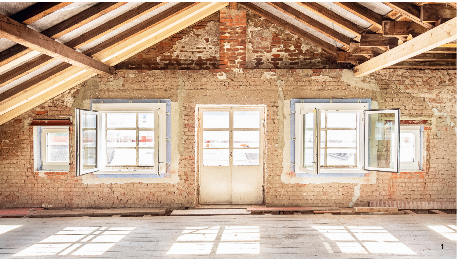
1 Combining the historic steel-framed windows on the outside with modern windows on the inside preserves the attractive appearance while providing effective thermal insulation. © Henning Krefit
