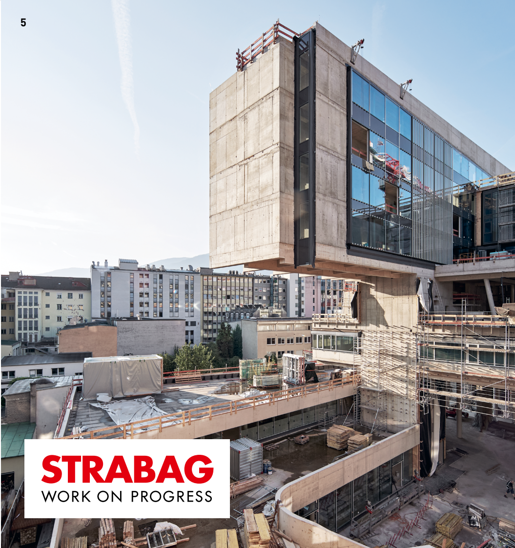
4 The location of the construction site in the centre of the city required sophisticated logistics planning. © STRABAG / Toni Rappersberger / 5 The „outstanding“ construction gives the hammerhead its name. © STRABAG / Toni Rappersberger
